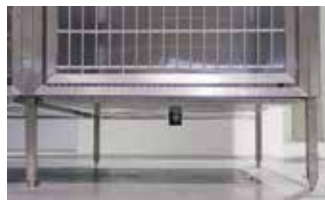
Stainless steel collection pan with nipple directs waste from each kennel to a central floor drain.
